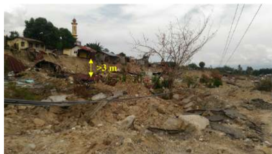
Figure 1.2. Road subsidence exceeding 3 m on the landslide crest caused by liquefaction in the Balaroa area.
