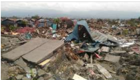
Figure 1.5. Damage caused by flow-type liquefaction phenomena.
