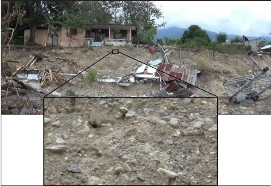
Figure 4.3.5. Lithological outcrop at the crown of the Balaroa landslide (Source: Buana, 2018).
