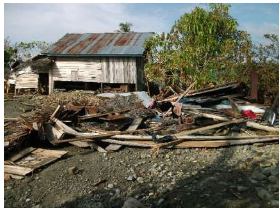
Figure 3.8. Tsunami trace at IAIN campus in Palu City with the flow depth of 1 m (left), and on Sirenja District, Donggala Regency with the flow depth 2 m (right).
